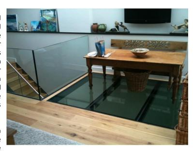
layers of 10mm glass with 2 no intermediate PVB interlayers. As the glass is supplied in a toughened speciation this glass retain no structural strength once broken and as such a sacrificial glass layer is provided so that should in the unlikely circumstance that one of the panes ever become broken then a full walk on specification unit is still provided.
